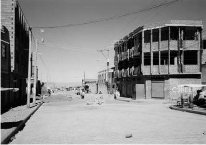
5. Work paving the central avenue in Rosas Pampa, Avenida 4, in 2000
